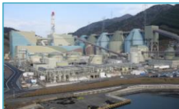
Maizuru Power Station (Coal fired power plant)
