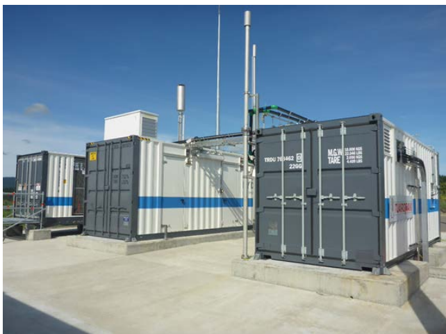
Power conditioner, Electrolyser, Gas compressor
