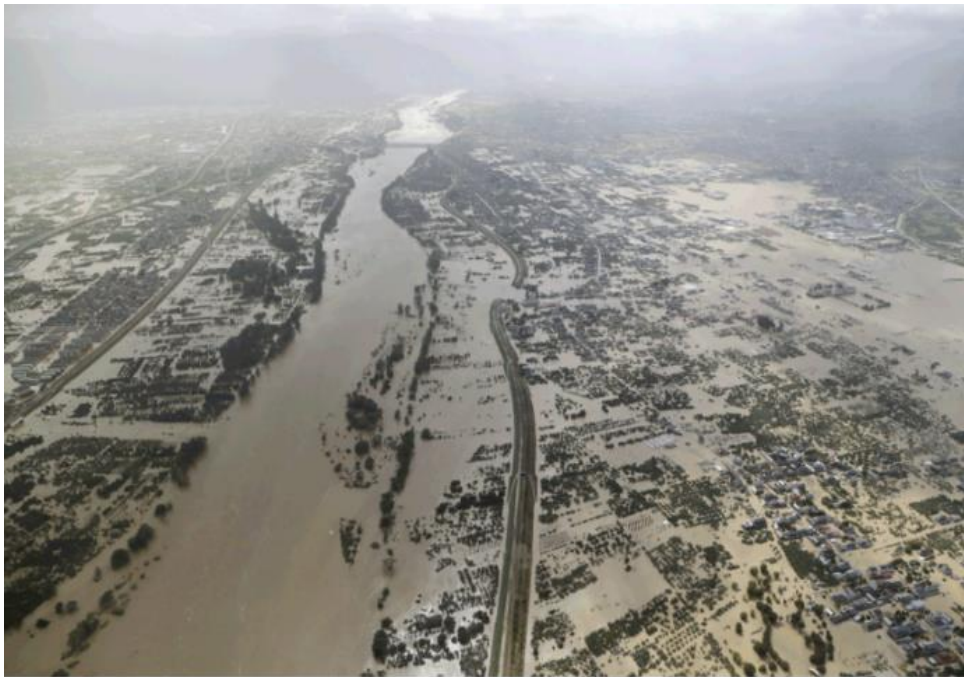
▲ Damage caused by Typhoon Hagibis in October 2019 <Chikuma River, Nagano City, Nagano Prefecture>
