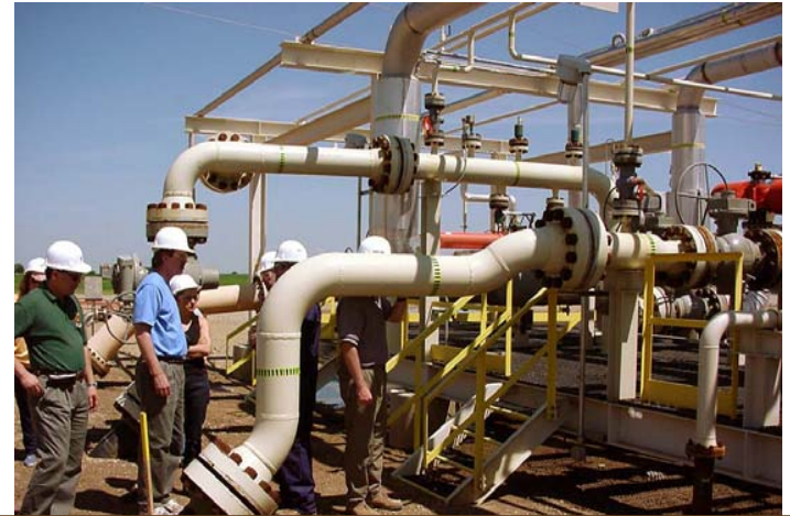
Main CO 2 pipeline enters Weyburn
