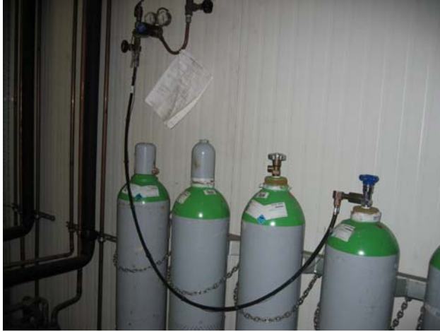
Fig. 6.14.1.2 – Ethylene station and cylinders
