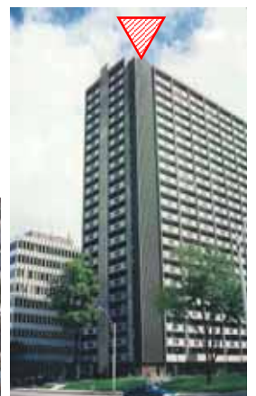
(写真提供 Conservall Engineering Inc.) 16
