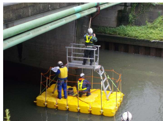
●浮き栈橋点検
