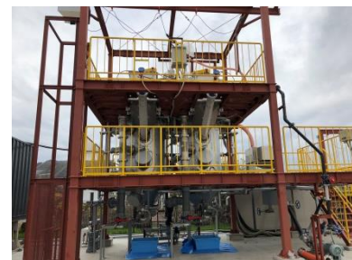
Methane fermentation tank
