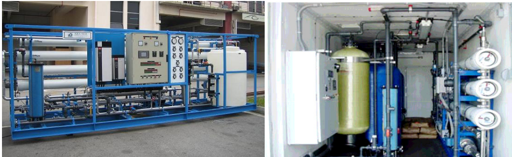
Figure 2-16 Integrated SWRO installed in a customized 20' ISO shipping container
