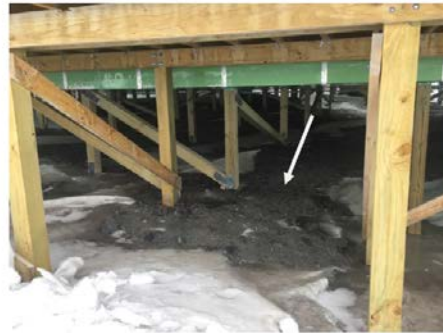
Visible ACM fragments under the Administration building
