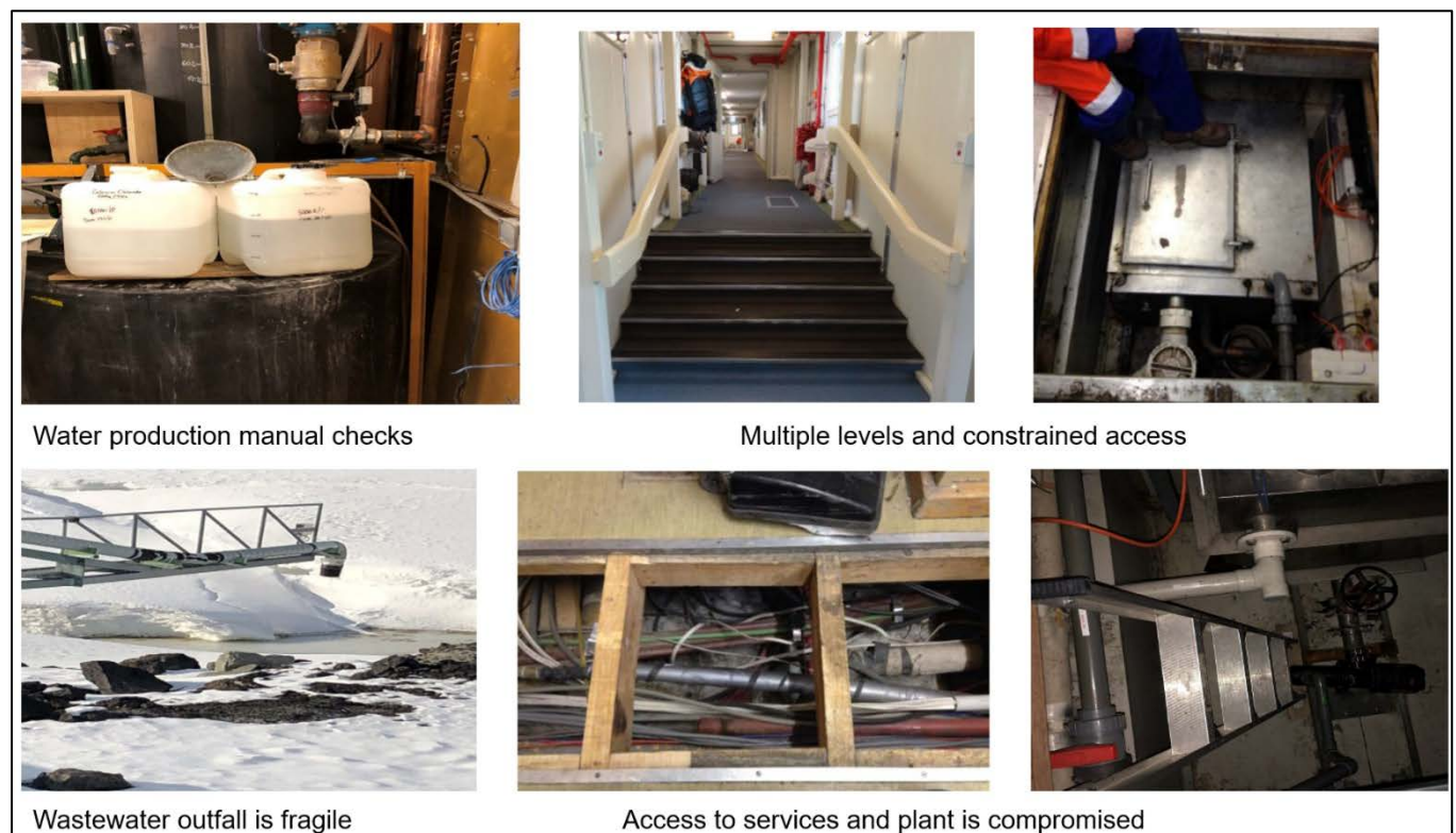
Figure 12: Examples of maintenance and infrastructure issues at Scott Base.
