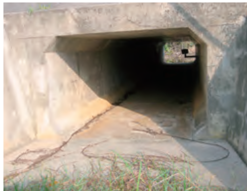
Example of improvement of road structure (adding an underpass) (Photo: JWRC)
