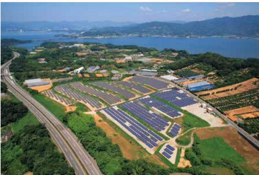
Hamamatsu Hamanako Solar Power Plant
