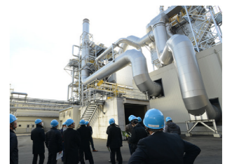
Wood biomass power generation plant
