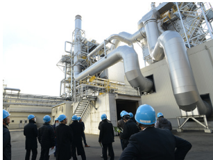
Wood biomass power generation plant
