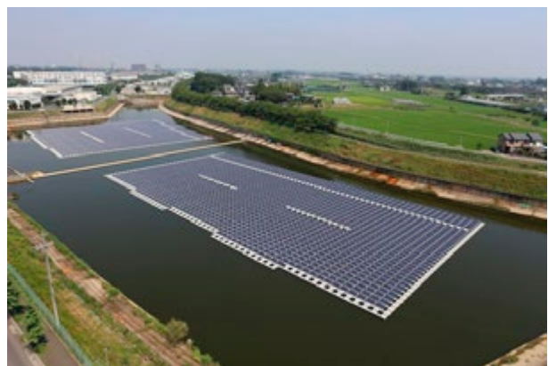
Floating megawatt solar plant in Okegawa
