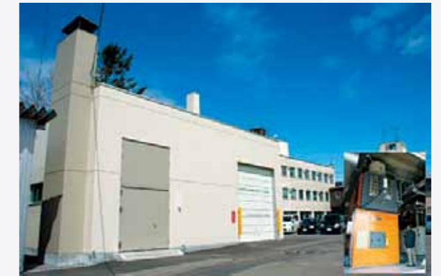
■Local heat supply center
