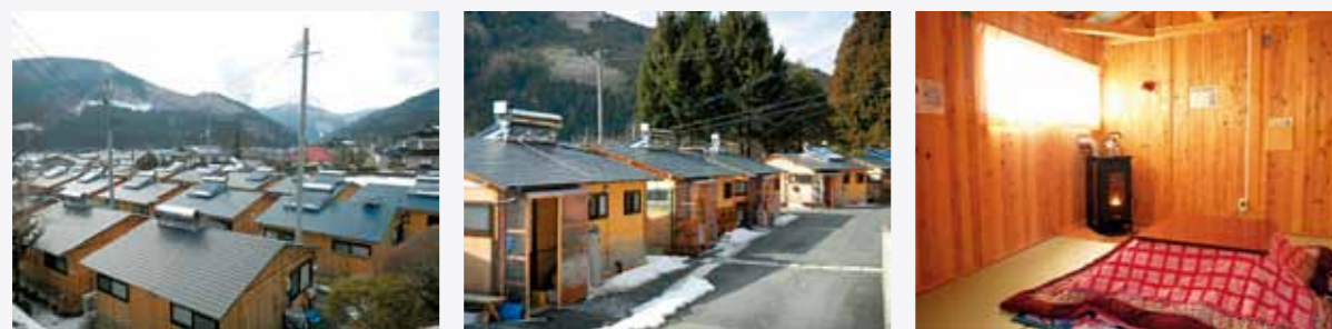
Temporary Housing Complex (bird's-eye view) Photos: Sumita Town
