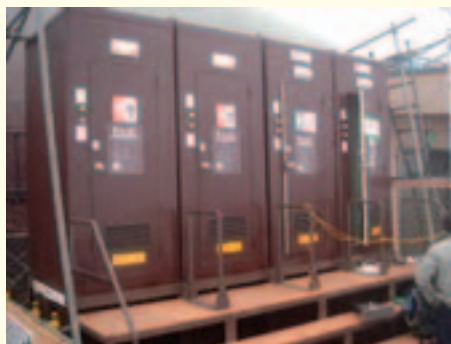
[Waste water treatment in mountainous areas] Source: Ministry of the Environment
