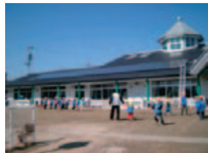
Day care center using solar power to generate electricity (Photo: courtesy of Iida City)
