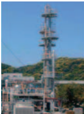
Overview of a long-term pilot plant for CO 2 capture (Photo: courtesy of Mitsubishi Heavy Industries, Ltd.)
