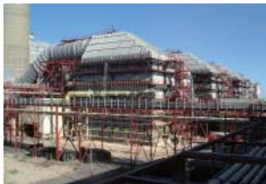
Flue gas desulfurization facility
