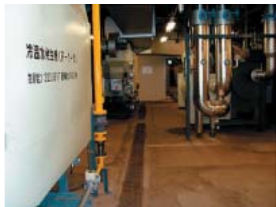
Turbo freezer and water chiller/heater
