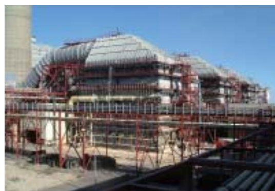
Flue gas desulfurization facility
