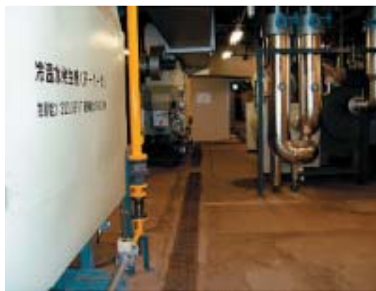
Turbo freezer and water chiller/heater
