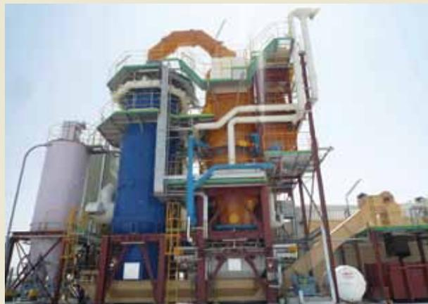
The medical waste incineration facility completed in Dubai is equipped with a vertical combustor that has the capacity to handle 19.2t/day and an air-purifying smoke and dust collection device for exhaust gas.
