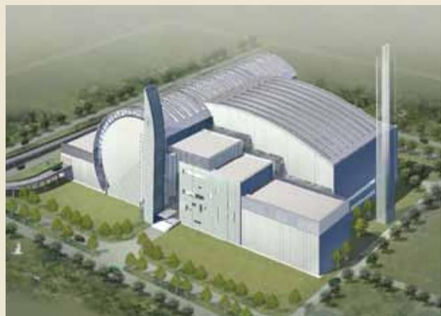
An electric generating facility with the capacity of 30,000 KW and steam condition of 4MPa and 400°C has been delivered to the incineration plant in Beijing, with capacity to handle 1,600t/day.
