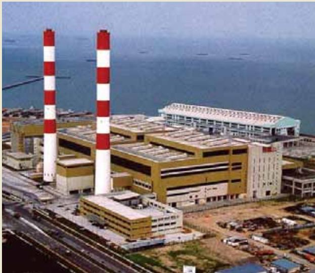
The largest scale plant with the capacity to handle 4,320t/day was built in Singapore in only 38 months
