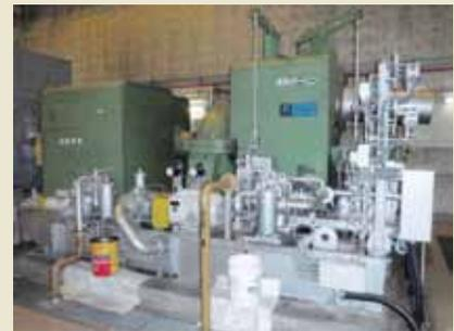
This incineration plant is equipped with a steam turbine generator that generates a maximum of 4,200kW, which is used in the plant. Excess electricity is sold to Tokyo Electric Power Company. The generator uses high-temperature water of 1Gcal/h, 130°C, with the maximum steam flow and pressure of 23.1t/h and 3.82MPa. (Shibuya Incineration Plant)
