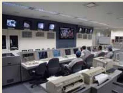
Operation of the incineration plant is managed from the central control room under automatic control (Shinagawa Incineration Plant)
