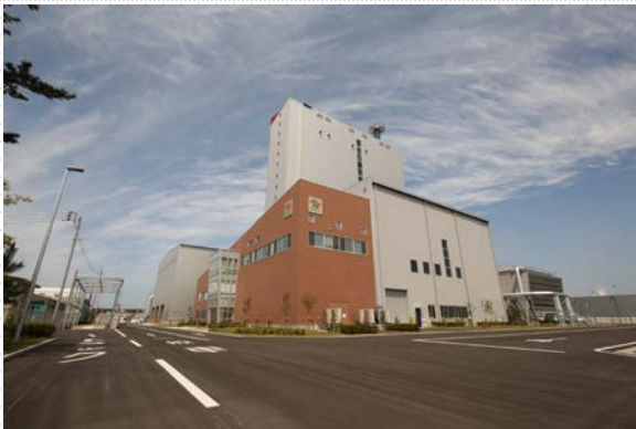
▲ Wood biomass power plant
