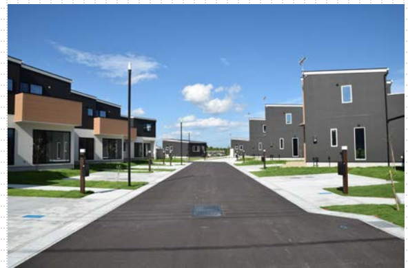
▲ Residential zone with no visible utility poles
