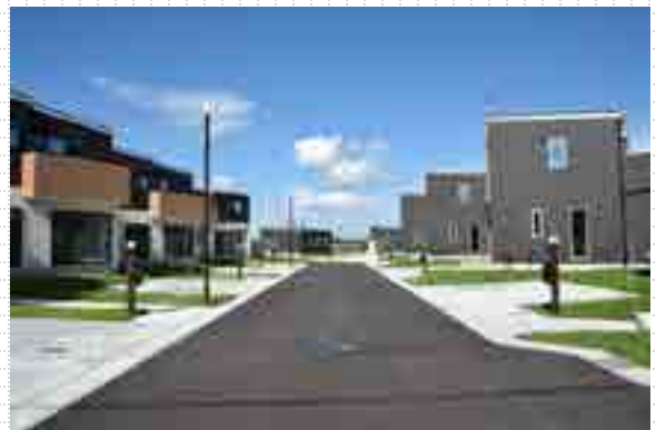
▲Residential zone with no visible utility poles
