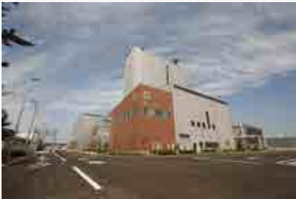
▲ Wood biomass power plant
