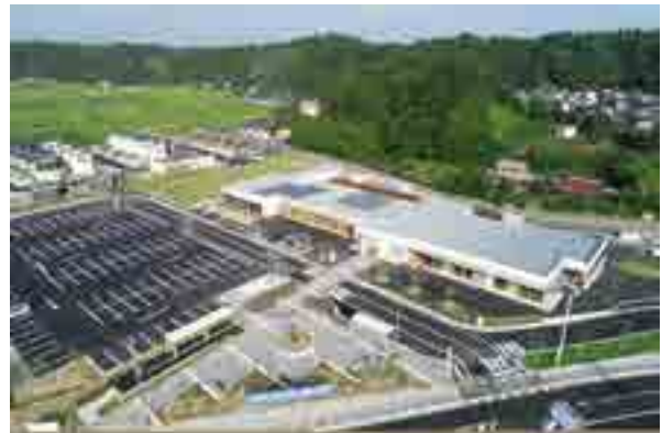
Mutsuzawa Smart Wellness Town (Mutsuzawa Tsudoi-no-Sato roadside station is in the foreground, with the residential area in the background.)
