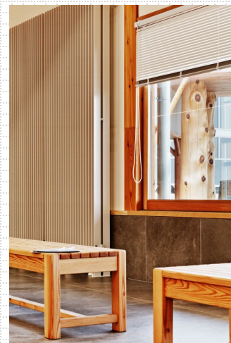
▲ Air-conditioning system using geothermal heat (Radiant panels)
