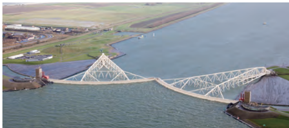
The Maeslantkering (movable storm surge barrier) in Rotterdam at the mouth of the Rhine. It protects the city from storm surges from the North Sea.
