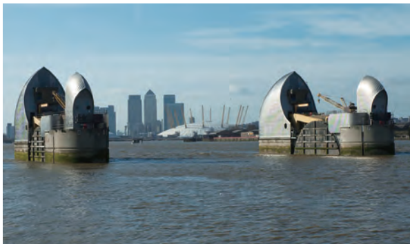
On the river mouth, the Thames Barrier is designed to protect inland areas from storm surges until 2030 even if sea level increases 8mm per year.
