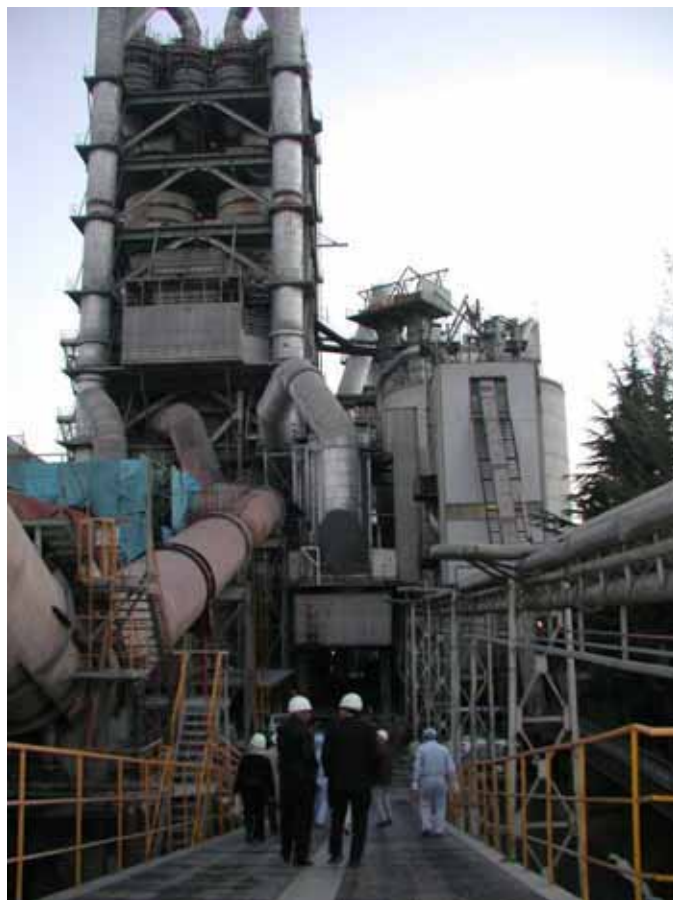
Figure 5.3-5 Cement Plant (Upper: Cement Kiln; Lower: Suspension Heater) (Chichibu Taiheiyo Cement. Japan)
