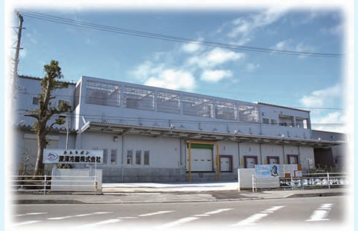
No. 2 Refrigerated Warehouse
