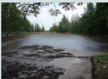
Anaerobic open lagoon on factory grounds (Ayutthaya Province, Thailand)
