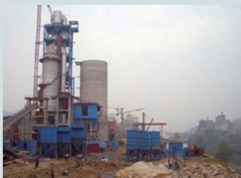
Dry rotary kiln under construction (Chongqing City, China)
