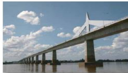
LAOS and THAILAND; Second Mekong International Bridge Construction Project
