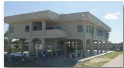
BANGLADESH; Construction of Multipurpose Cyclone Shelters Project V
