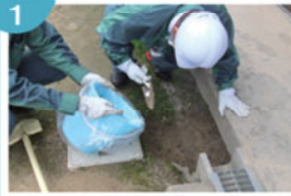
●民家の軒下・雨樋の清掃
