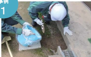
●民家の軒下・雨樋の清掃
