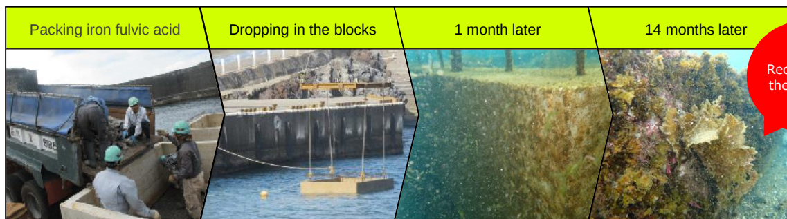
Dropping the blocks in the sea, and observing the restoration process
