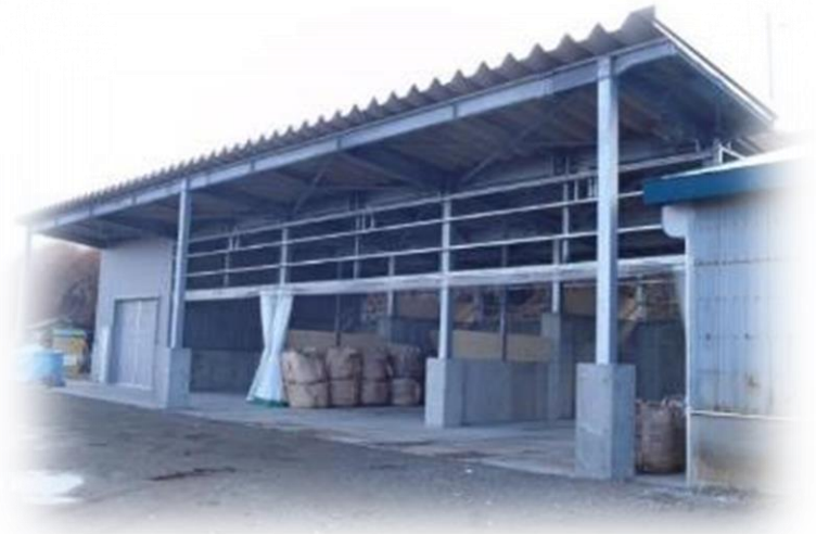
In-house-built compost production facility
