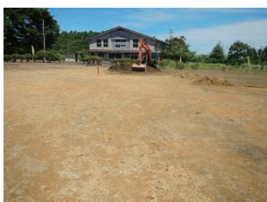
Decontamination work at Ono Kindergarten in Okuma Town
