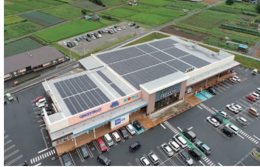
Commercial facility with solar power generation system Source: i GRID SOLUTIONS
