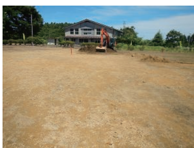
Decontamination work at Ono Kindergarten in Okuma Town
