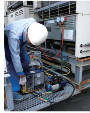
Recovery of refrigerant from super-market cold showcase Source: Refrigerants Recycling Promotion and Technology Center, Japan
