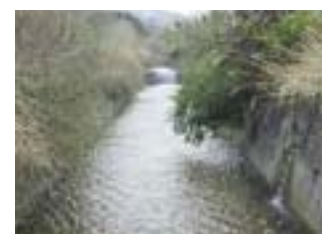
Channelized concrete canal in the wetlands
