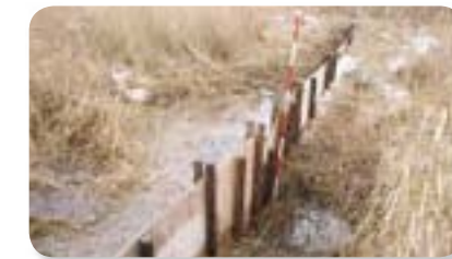
Immediately after damming, at the outflow of Ochiai-numa Pond (the dike is 10.5-m long and 1.1-m high above the ditch bottom).
