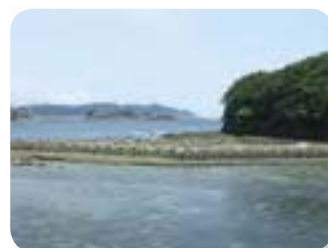
An existing breakwater levee
