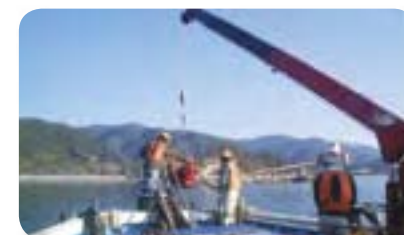
A small-sized crane and dredge pump
