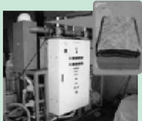
(直接加熱法)吸着回収装置 [予定]
