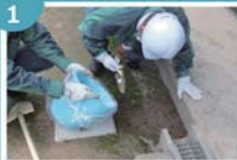
●民家の軒下・雨樋の清掃
