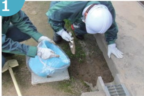
●民家の軒下・雨樋の清掃
