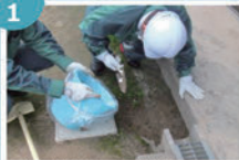
●民家の軒下・雨樋の清掃
