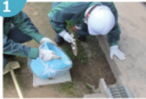
●民家の軒下・雨樋の清掃
