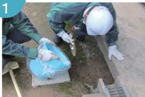
●民家の軒下・雨樋の清掃
