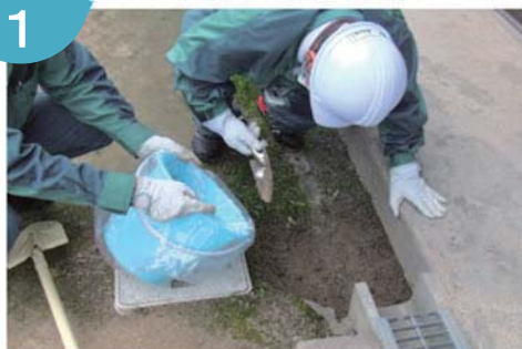
●民家の軒下・雨樋の清掃
