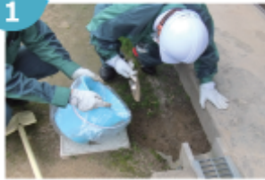
●民家の軒下・雨樋の清掃
