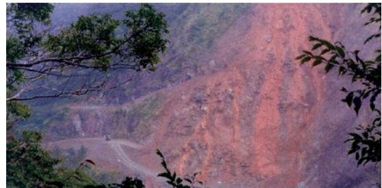
Photo 4. Red soil is exposed due to development activities (Amami Oshima)
