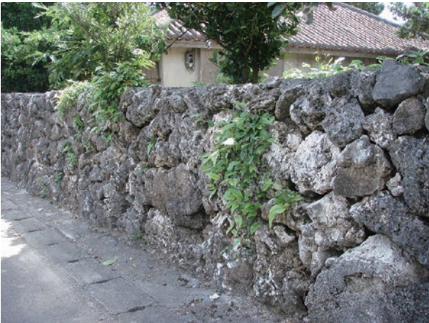
Photo 16. Stonework made of Ryukyu limestone and coral seen in Shiraho Village (Provided by WWF Japan)
