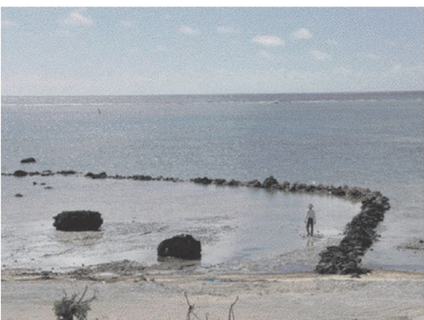
Photo 18. Restored inkachi (Provided by WWF Japan)
