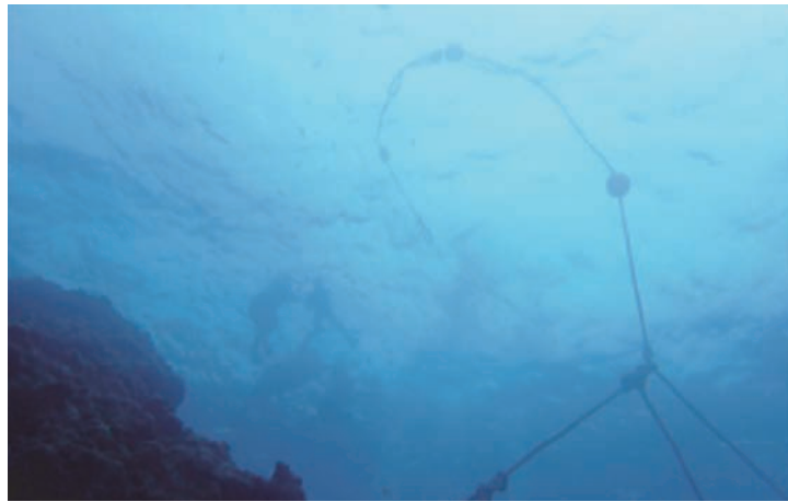
Photo 11. An Anchor buoy set up in the marine areas in Maedamisaki (Onnason)
