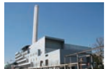
State-of-the-art equipment for the prevention of pollution, including dioxin emission control, was introduced in the Chitose Waste Processing Factory completed in March 1996.
