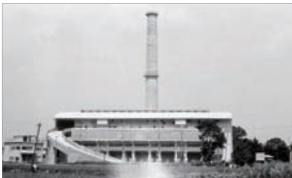
The Fifth Waste Treatment Plant constructed in Tokyo in 1958 was equipped with six large incineration furnaces and was built based on new design concepts. The plant was designed to dry garbage and other waste containing large amounts of moisture and was equipped with a system that transported waste incineration ash by using belt conveyors. It also provided hot water supply services to local communities using residual heat.
