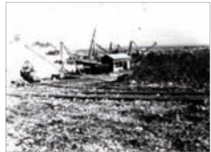
Landfill on Dream Island in Tokyo Bay. Most of the waste was not incinerated or covered with soil, generating problems such as spontaneous combustion caused by garbage fermentation gases, as well as foul odors and plagues of flies.
