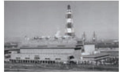
Constructed in Tokyo in 1973, the Oi Waste Processing Factory contributed to solving waste problems as a large factory equipped with bulky waste crushers and waste reloading devices. The factory supported the design of incineration furnaces and the improvement of facilities required to cope with changes in the quality of waste as well as with the collection of bulky waste.
