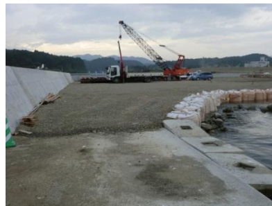
Shizugawa fishing port south-side breakwater restoration work
