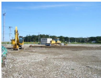
Reconstruction work in Yamamoto Town, Miyagi Prefecture
