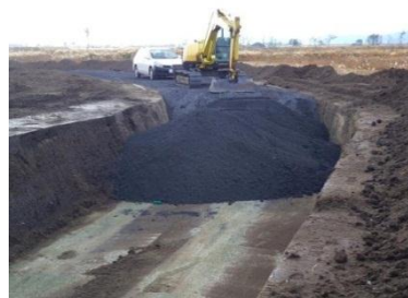
Cycling road construction work in Natori town, Miyagi pref.
